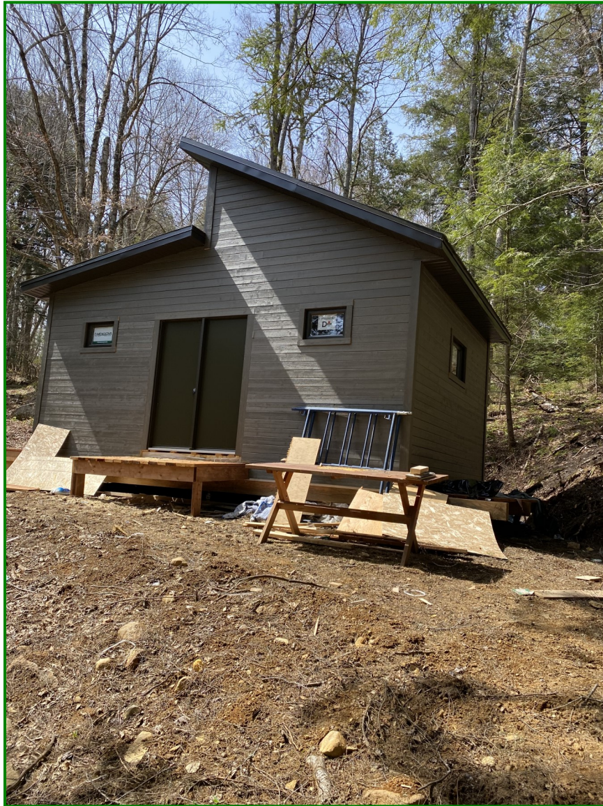
Picture of the new bath room /shed on Goulden Island
